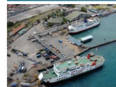
Merak Ferry Terminal
