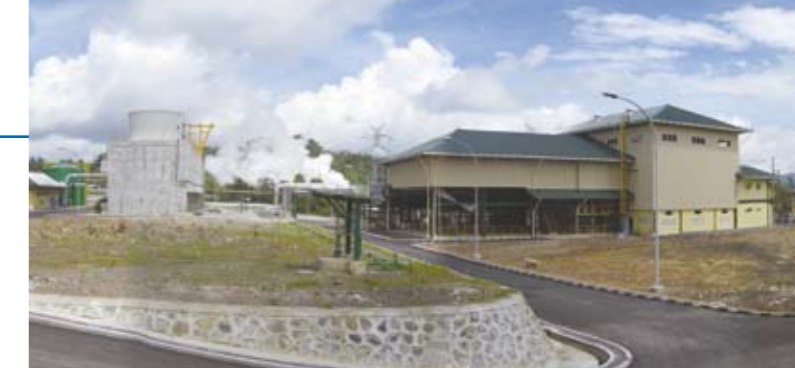
Lahendong Geothermal Plant
