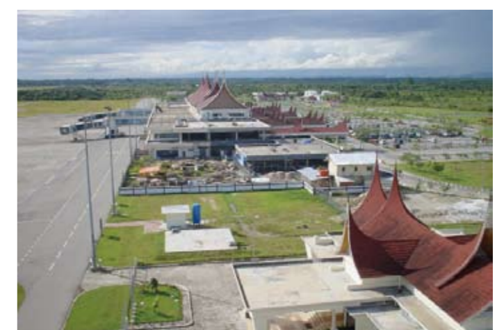
Minangkabau Airport (Padang)
